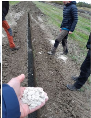
Filter ditch with lime
