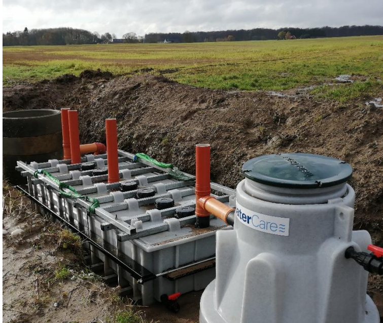
Figure 2. Dual porosity filter (DPF) unit, WaterCare Filtration A/S, with flushing pipes extending vertically and inspection well installed at the Fensholt site.
