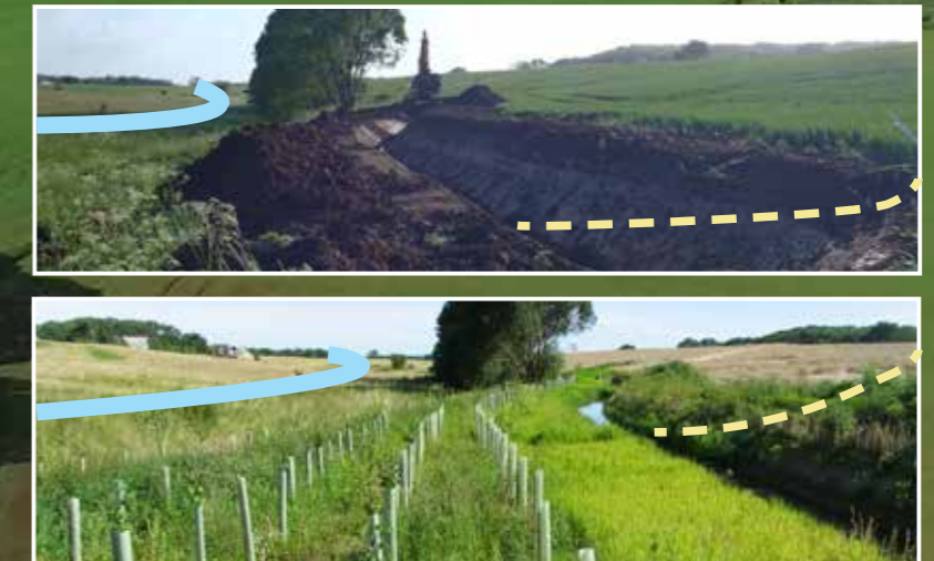
Integrated buffer zone at Odder. The blue lines represent the stream and the yellow dotted line is the drainage inflow.
